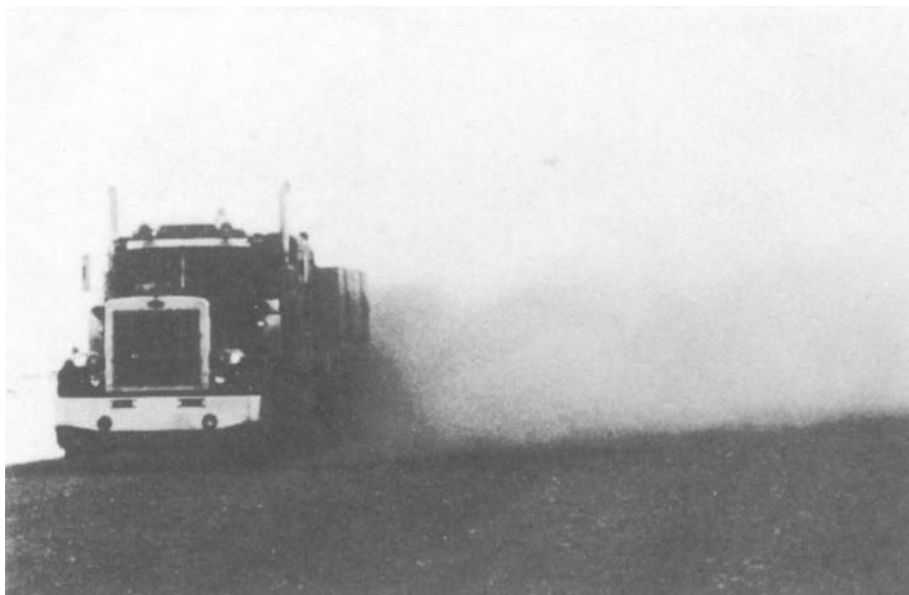
Figure B-8. High severity example of dust.
